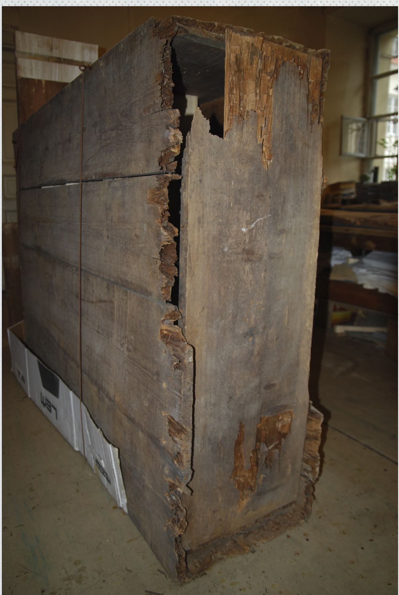
ill. 2. Before restoration.
