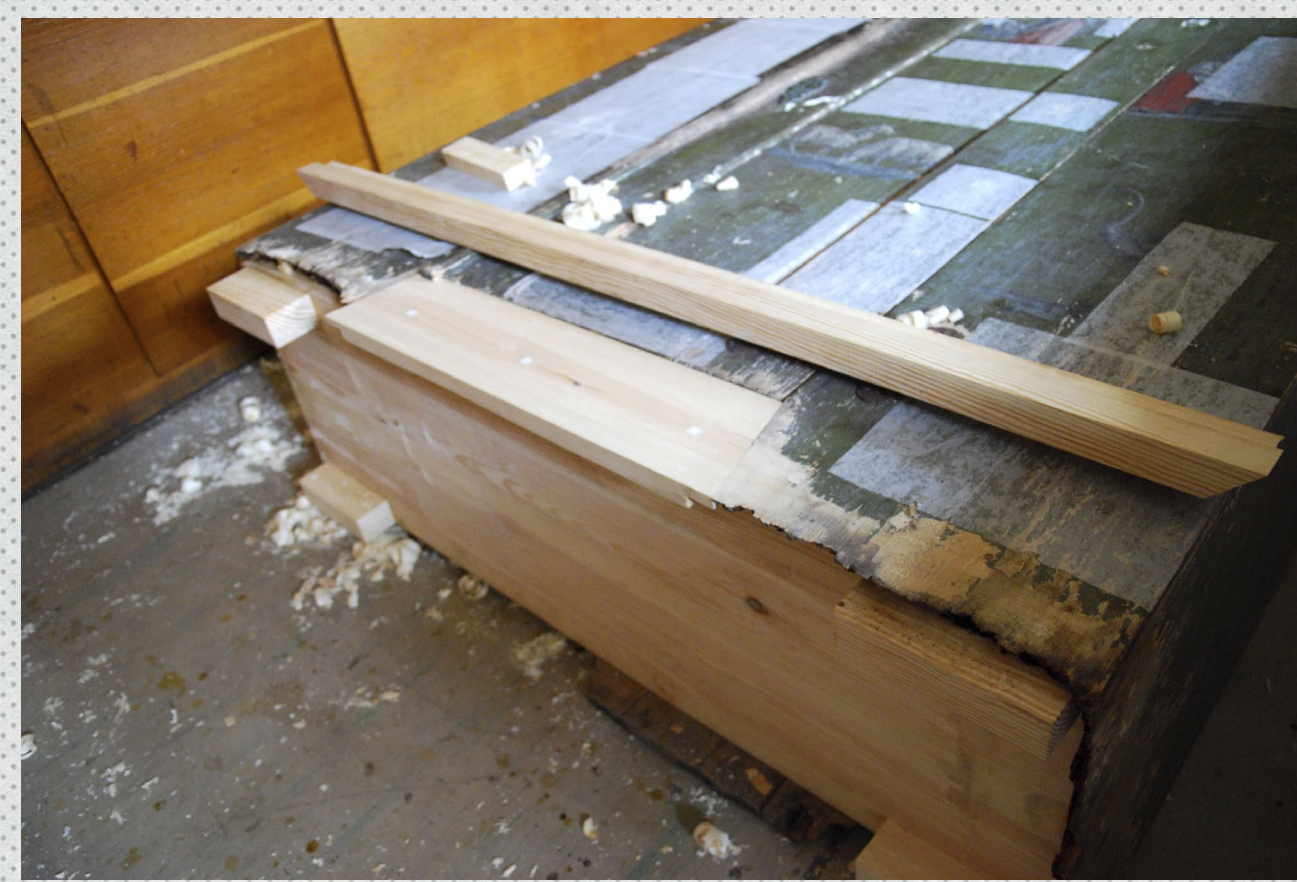
ill. 3. During restoration. Reconstruction of the sideboards.
