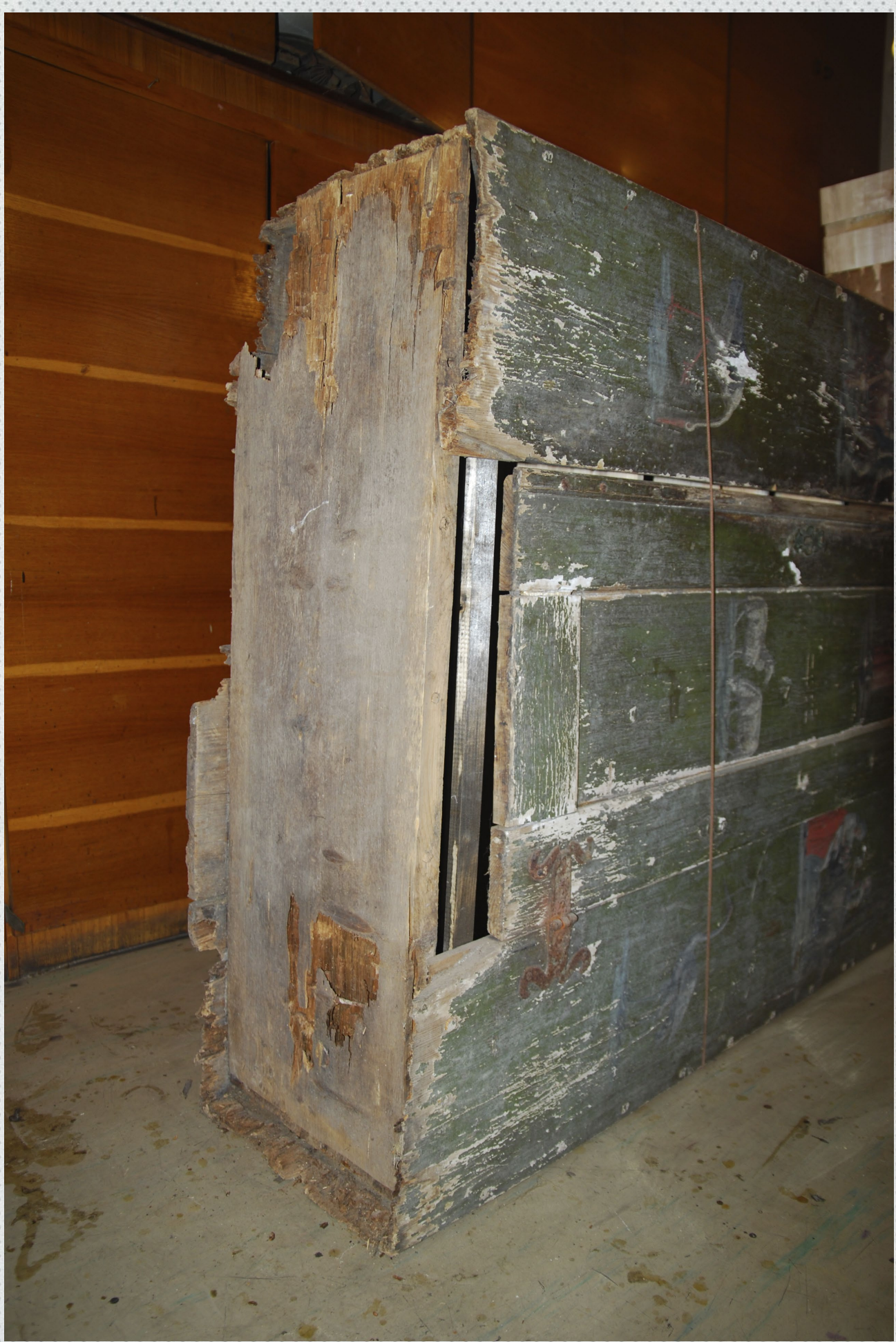
ill. 1. Before restoration.
